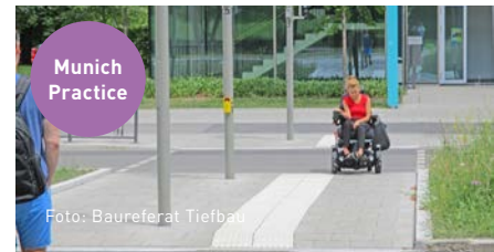
SEPARATE CROSSINGS, Munich In a pilot project, a separated crossing point with differentiated curb height (0 / 6 cm) was implemented for the first time in 2022 to meet the needs of blind and walking-impaired people.
