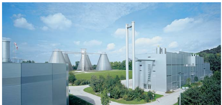
The sludge incineration plant together with the completed sludge digesters (composite photo).
