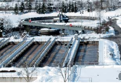
The Wastewater Treatment Plant Gut Großlappen is equipped with a mechanical and two biological treatment stages. Samples are taken systematically from all treatment stages and analysed in the plant's own laboratory.
