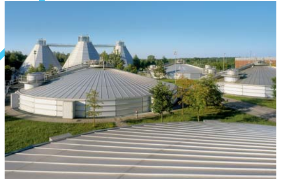
Wastewater Treatment Plant Gut Marienhof
