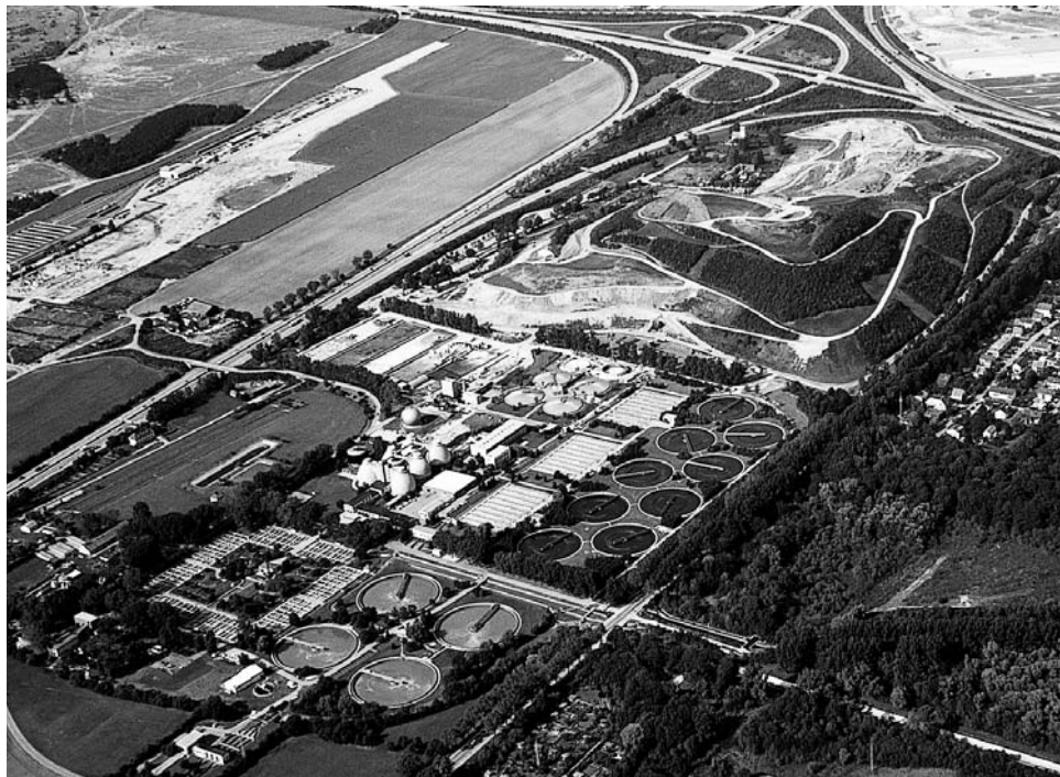
2006: Construction of new sludge digesters and an effluent sand filter
