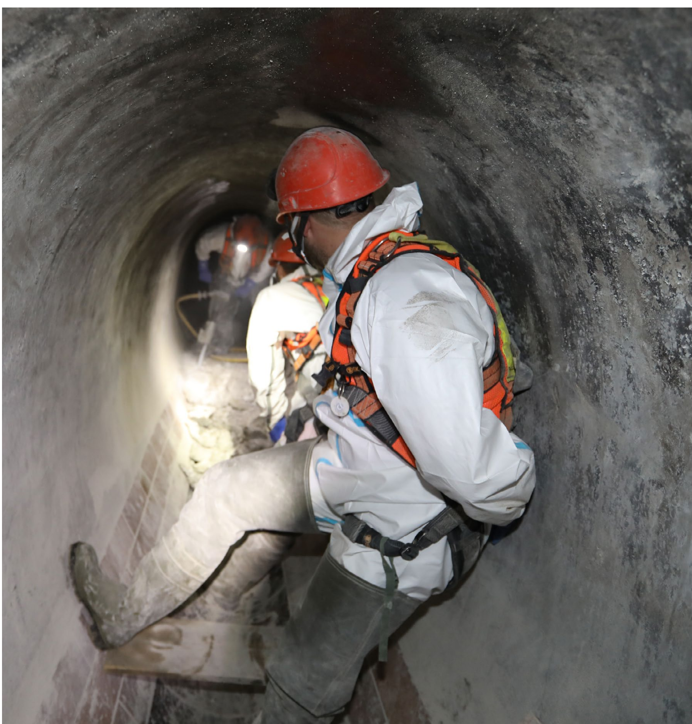
MSE employees remove concrete with a demolition hammer
